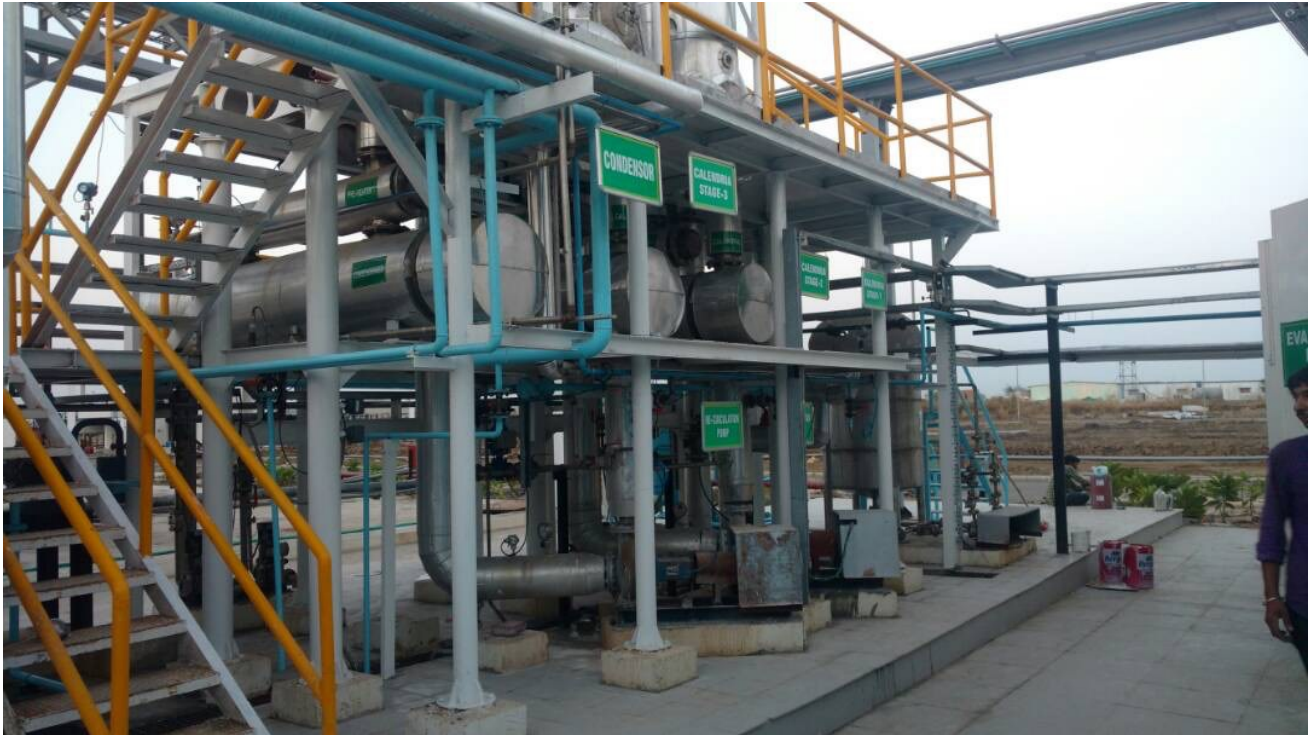
Above: A zero liquid discharge system is being proposed for water desalination. https://upload.wikimedia.org/wikipedia/commons/3/3a/Zero_liquid_discharge_system.png
